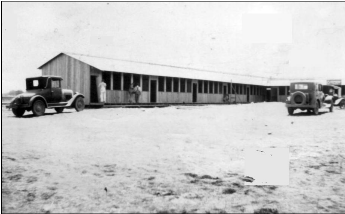
Figure 4. View of Grant Union High School, ca. 1932, showing six of the facility’s 16 temporary classrooms (Photograph courtesy of the Grant Union High School Alumni Association, Sacramento).
