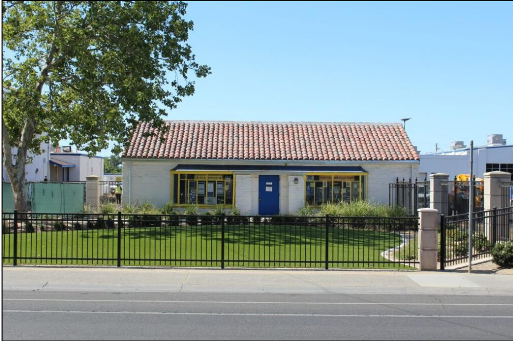
Photograph 15. View of the north (front) façade of the School Store, facing south (H. Fuess, 2025).
