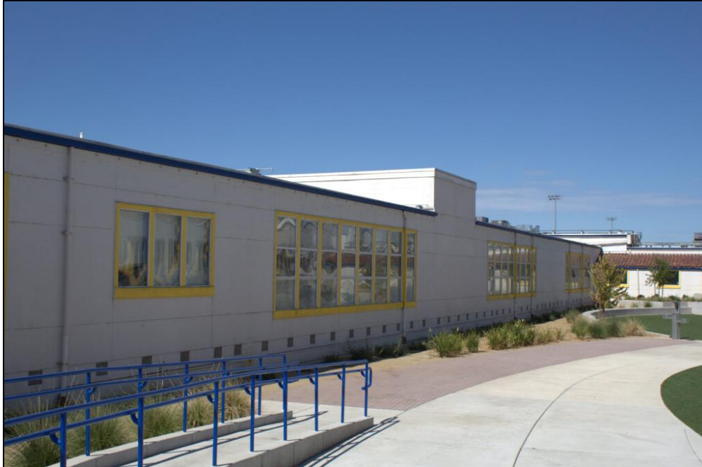
Photograph 11. View of the north (front) façade of the 1939 addition to the Main School Building, facing southwest (H. Fuess, 2025).
