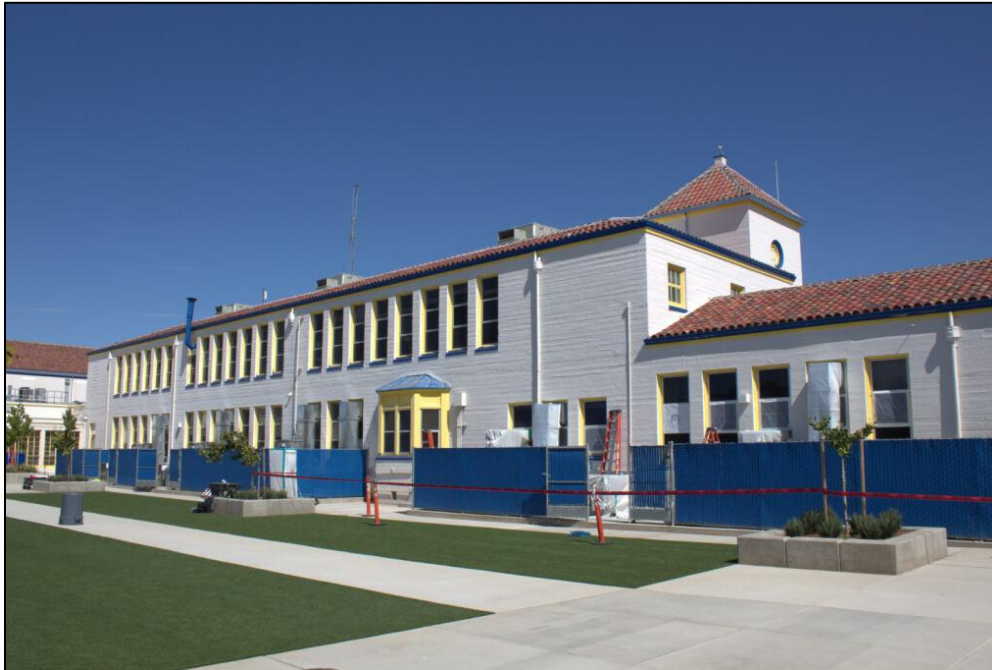
Photograph 7. View of the south (rear) façade of the 1935 portion of the Main School Building, facing northwest (H. Fuess, 2025).
