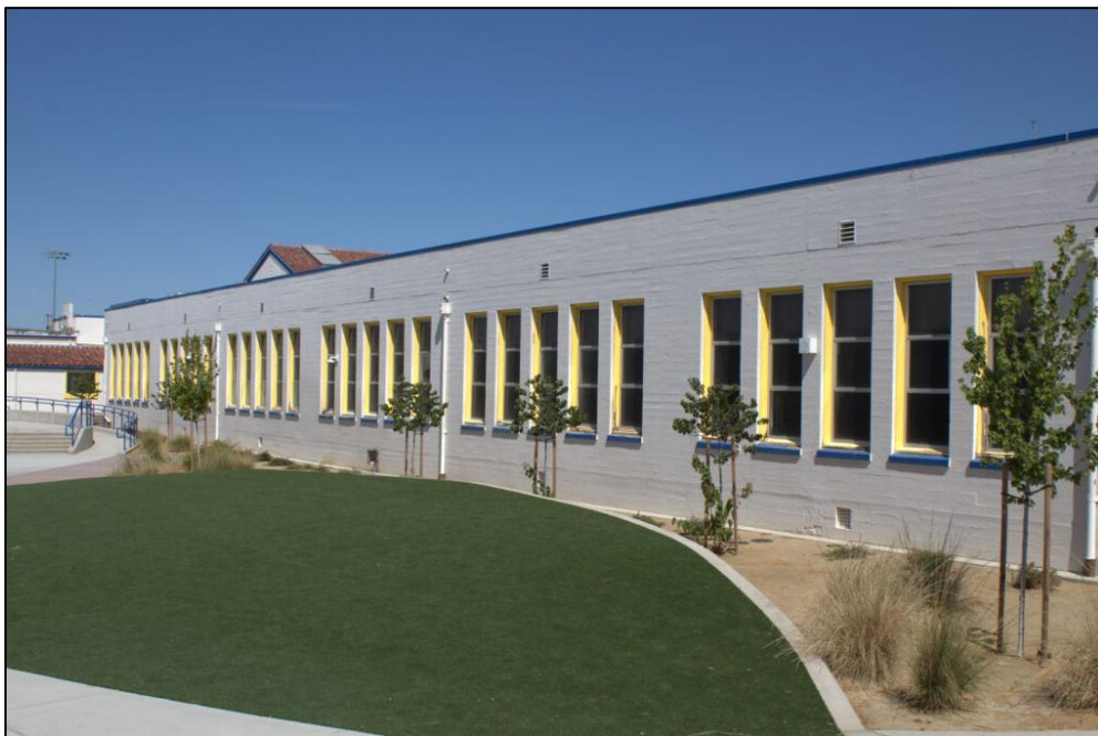
Photograph 10. View of the south (rear) façade of the 1937 addition to the Main School Building, facing northwest (H. Fuess, 2025).
