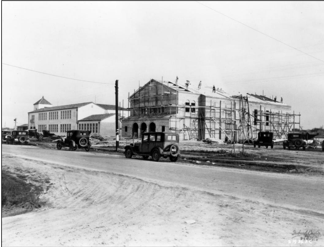
Figure 6. View of auditorium under construction, ca. 1935 (Photograph courtesy of the Grant Union High School Alumni Association, Sacramento).
