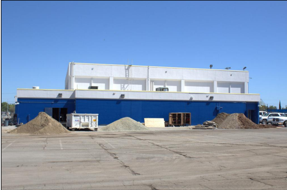
Photograph 23. View of the west (front) façade of the Gymnasium, facing east (H. Fuess, 2025).
