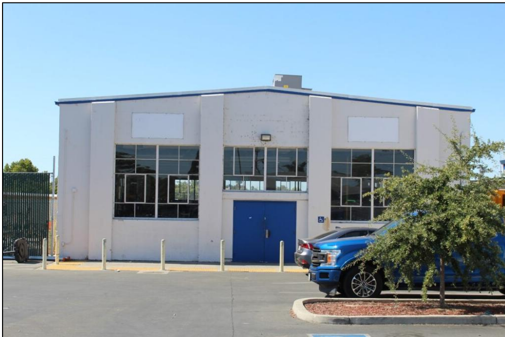
Photograph 20. View of the north (front) façade of the Shop #3, facing south (H. Fuess, 2025).
