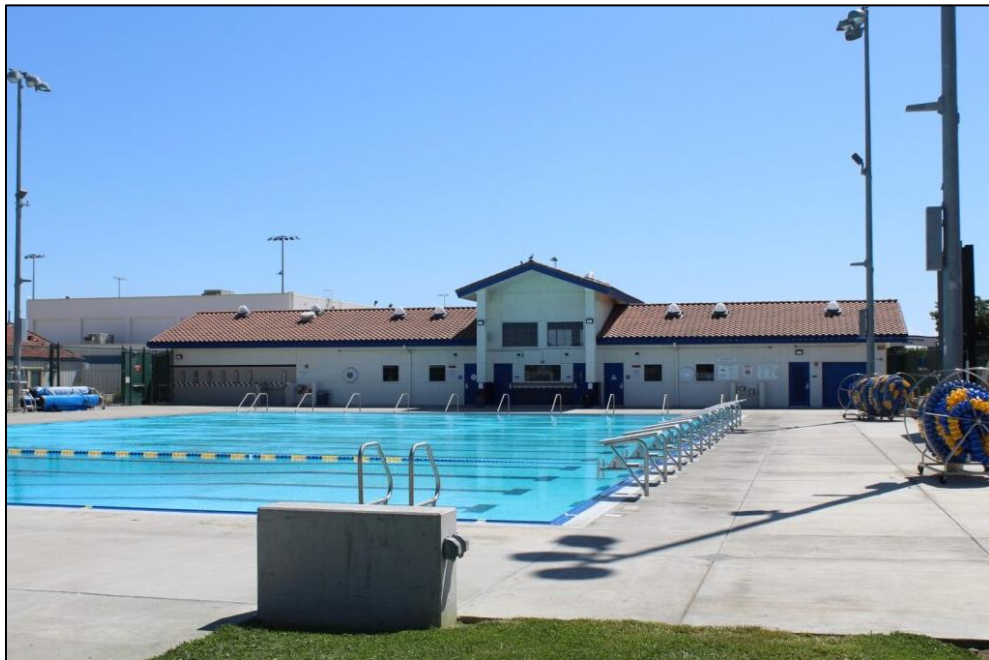
Photograph 24. Overview of the Swimming Pool and Pool House, facing east (H. Fuess, 2025).
