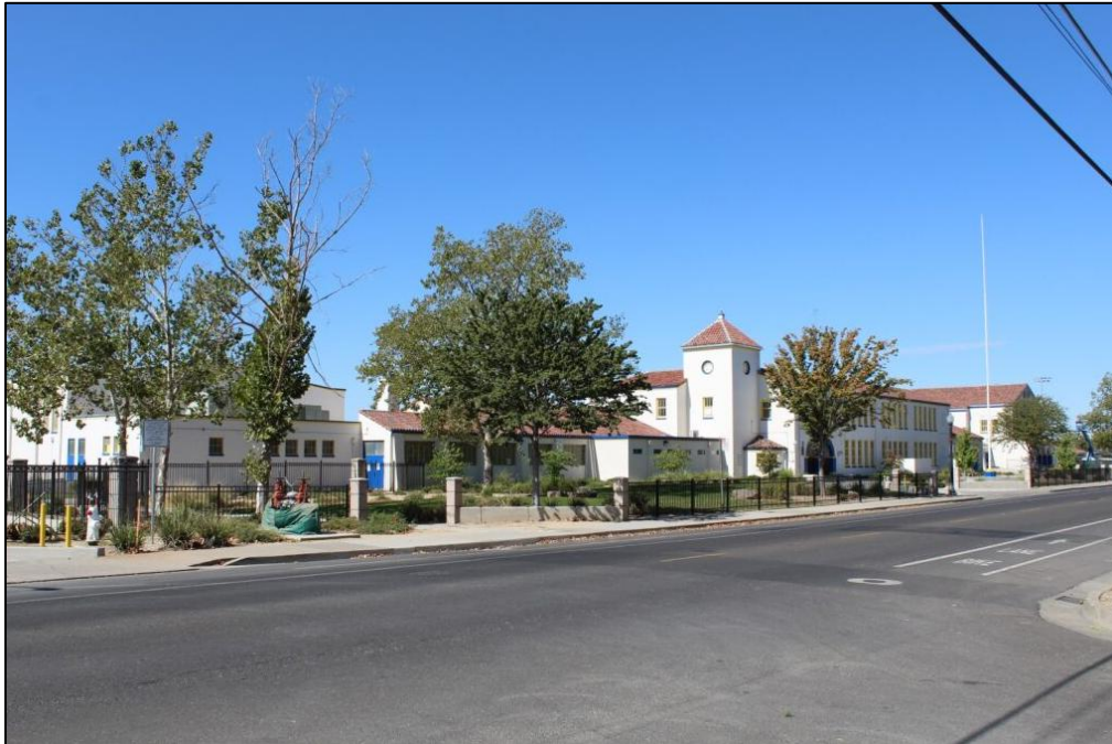
Photograph 1. Overview of Grant Union High School, facing southwest (H. Fuess, 2025).
