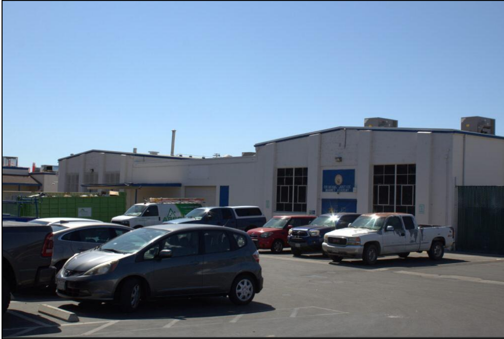
Photograph 17. Overview of Shop #1 and Shop #2, facing southeast (H. Fuess, 2025).
