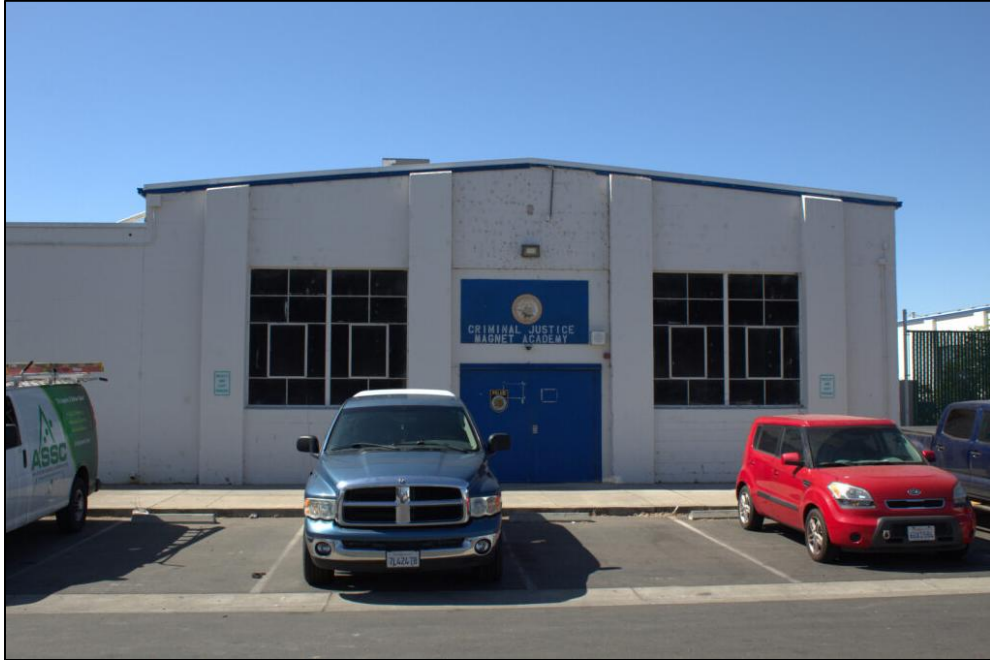
Photograph 19. View of the north (front) façade of the Shop #2, facing south (H. Fuess, 2025).
