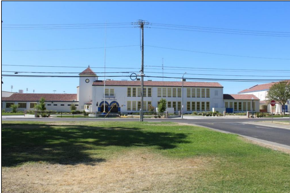
Photograph 5. View of the north (front) façade of the Main School Building, facing south (H. Fuess, 2025).
