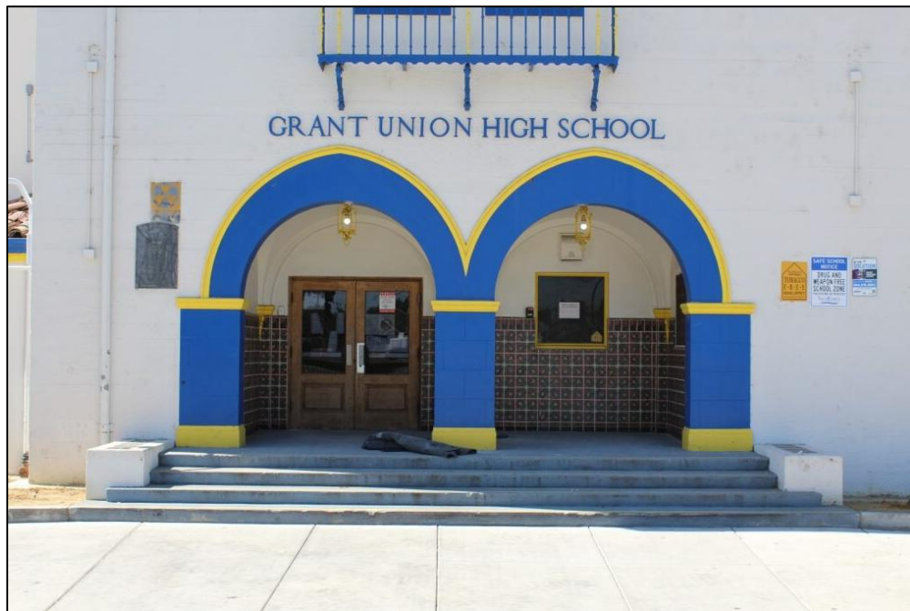
Photograph 6. Detail view of the front entrance to the Main School Building, facing south (H. Fuess, 2025).
