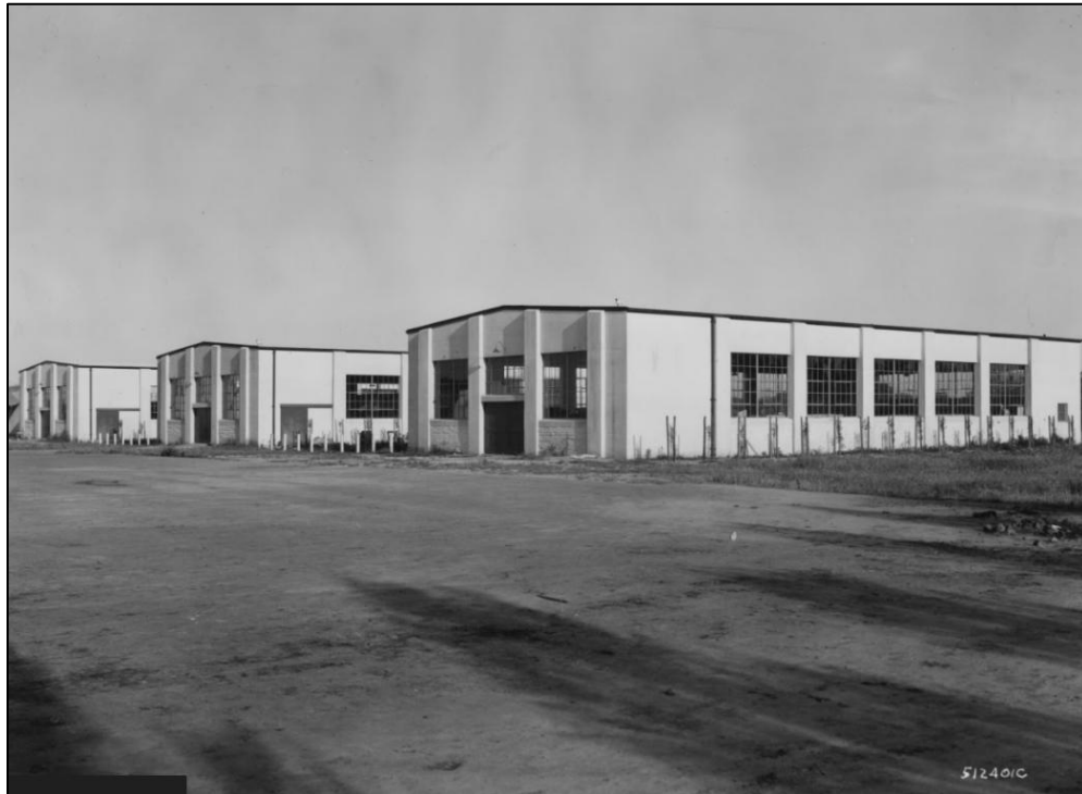
Figure 10. Overview of the completed shop buildings, ca. 1939 (Photograph courtesy of the Grant Union High School Alumni Association, Sacramento).
