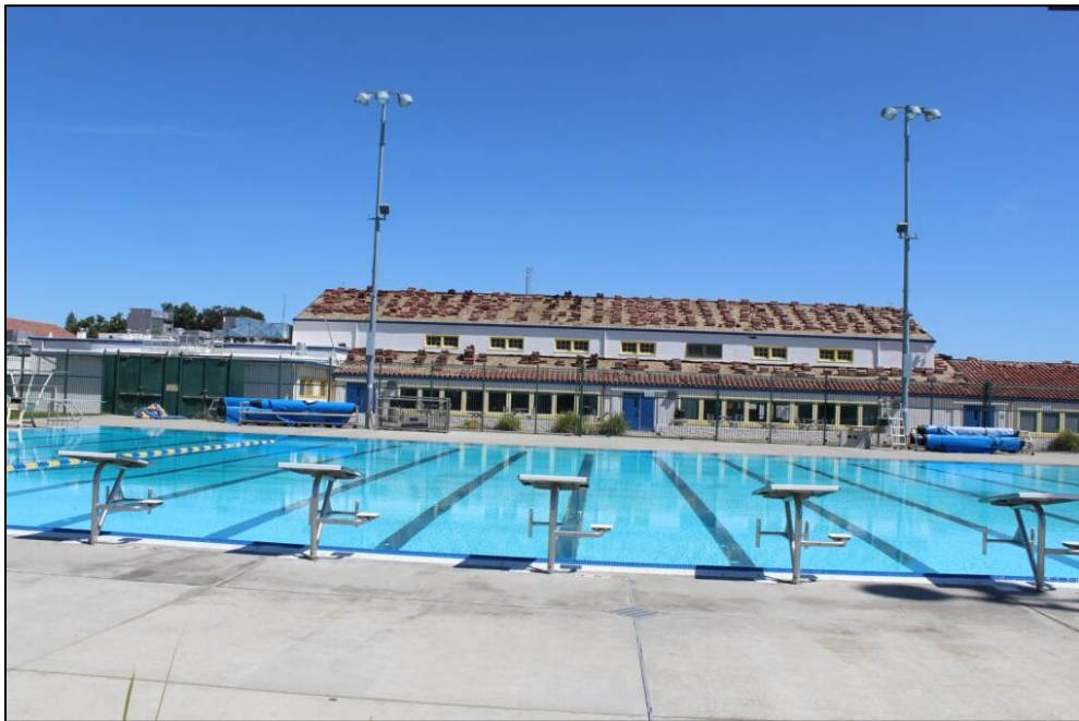
Photograph 22. View of the south (front) façade of the Cafeteria, facing north (H. Fuess, 2025).
